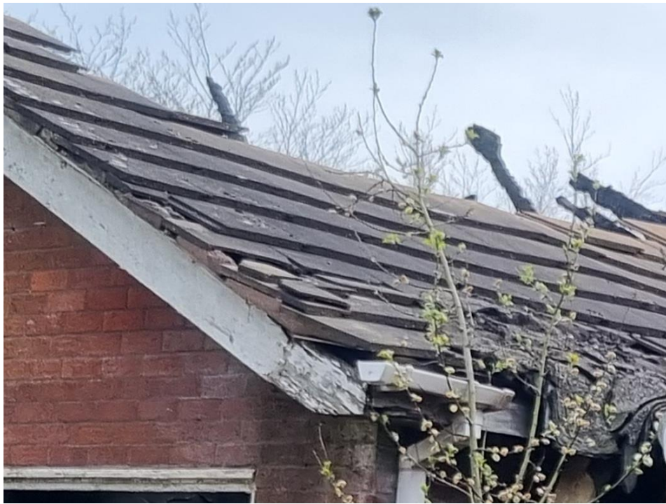
Photograph 3: Remaining section of dwelling roof with inter-locking concrete tiles
