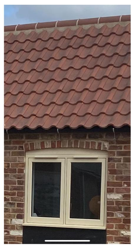
As per the planning application the Windows will be a cream-coloured uPVC casement windows of multiple sizes to allow for adequate ventilation and means of fire escape.
