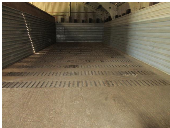
Photograph # 8 (Typical Raised 'Drier' Floor)
