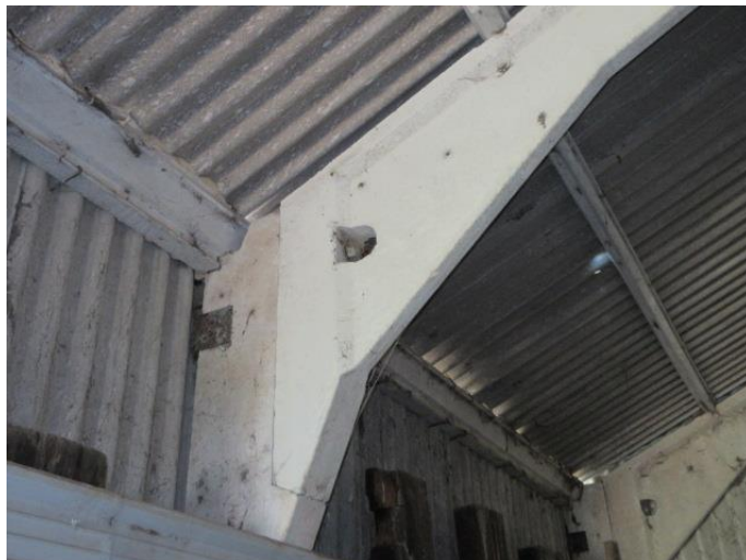
Photograph # 6 (Typical Existing Frame– Eaves Haunch )
