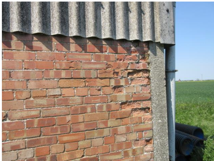
Photograph # 11 (Typical External Brickwork – Isolated areas of defaced masonry)
