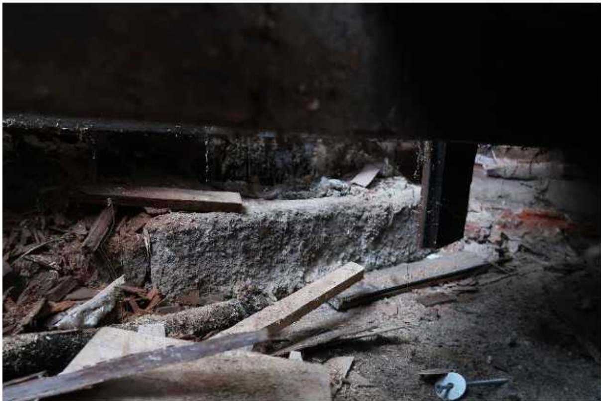
Image H: The oak wall-post footing stone, also showing the sub-floor void and sleeper wall
