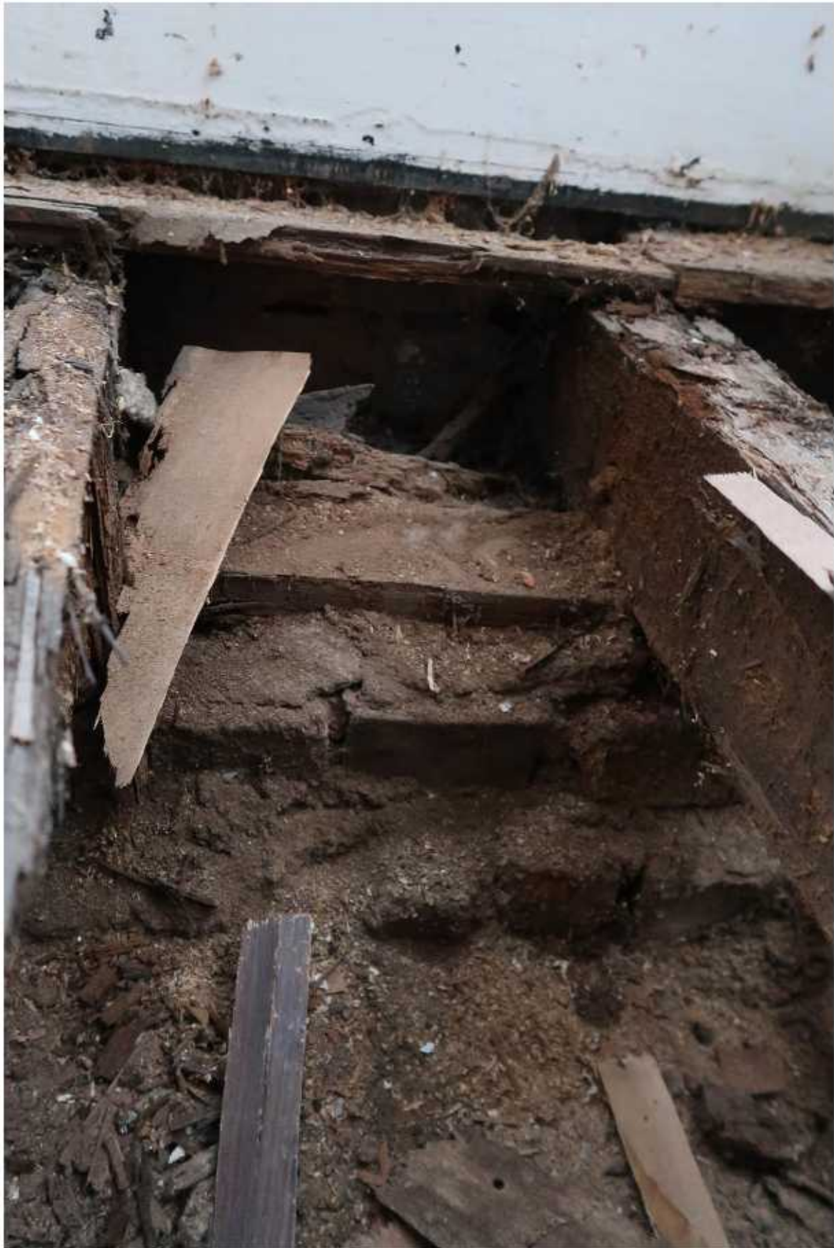
Image F: The joist bearer damaged by wet rot, laid onto the brick plinth wall
