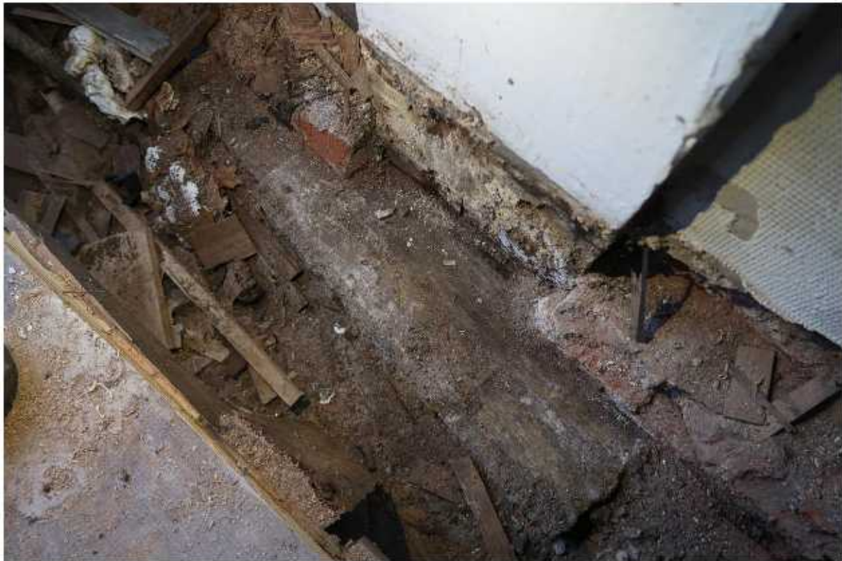
Image G: The oak wall-post footing stone in the sub—floor void
