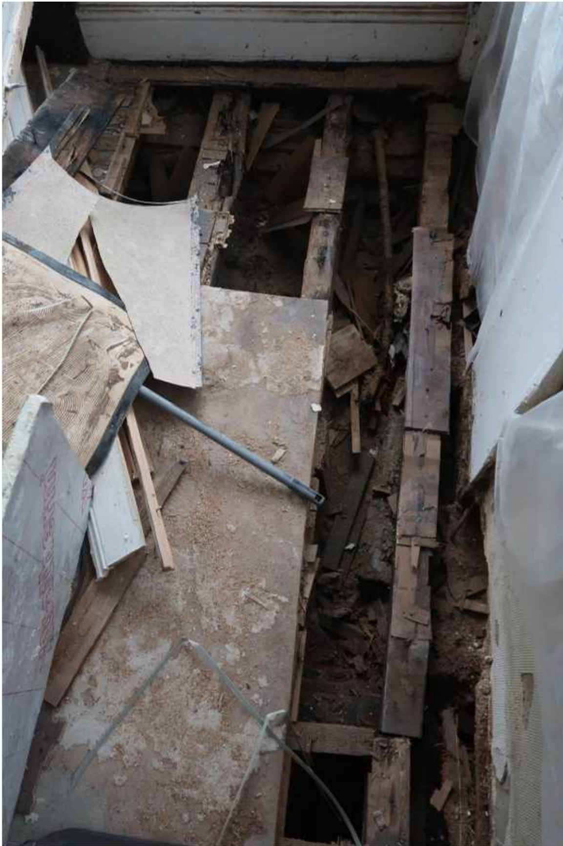
Image C: The exposed floor structure – Boards and plywood are lifted showing the joists and void
