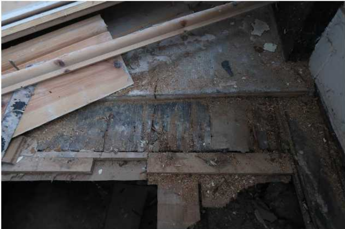
Image D: The earlier floorboards exposed, with later softwood patching visible.
