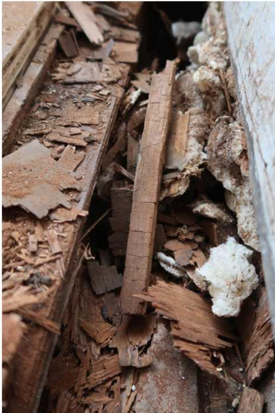
Image A: during removal of the floorboards, showing rotten existing boards (NB - the white foam on the right is expanding foam insulation)
