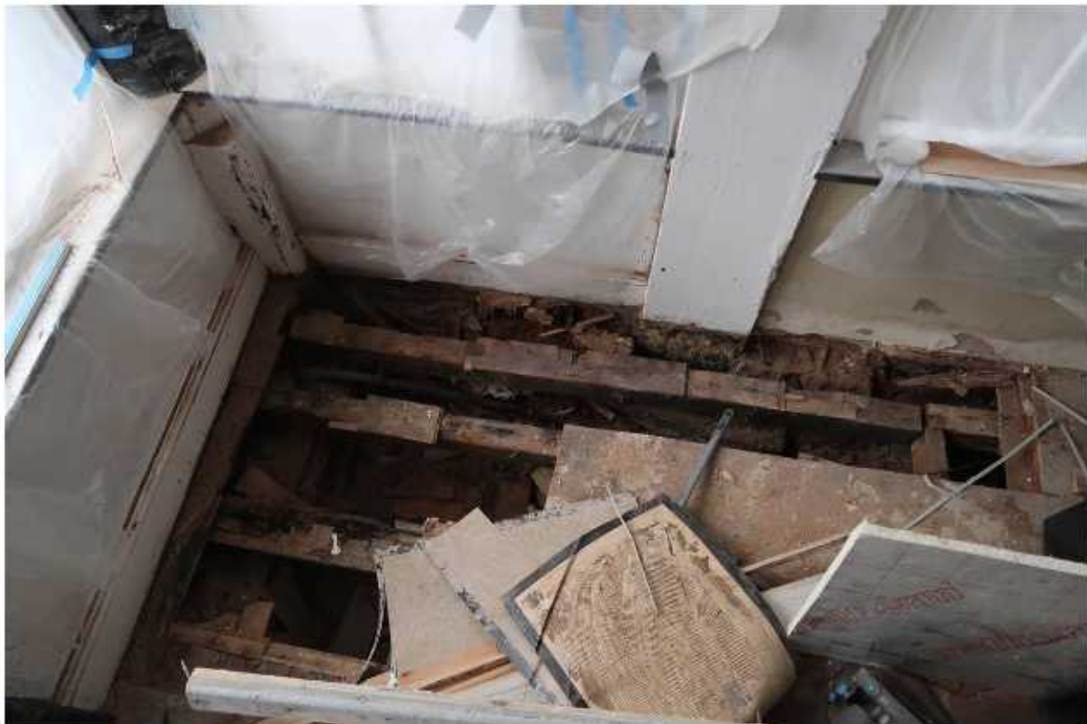
Image B: The area of exposed floor structure – the boards and plywood are lifted
