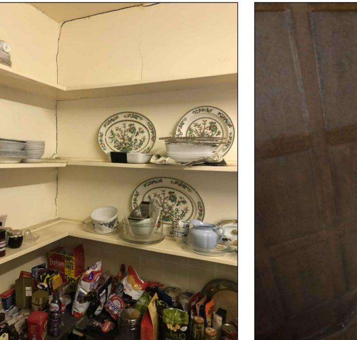
Cut back render on brick/block wall to a min 75mm either side of cracking. Carefully rake out fractured mortar bed joints. Wedge and repoint using a 1:1:6 cement lime sand mortar, colour and texture to match existing as far as is reasonably practical. Supply and fit Expamet mesh and render, including applying PVA bonding agent, to match existing pattern and texture as far as is reasonably possible fixed to brick
